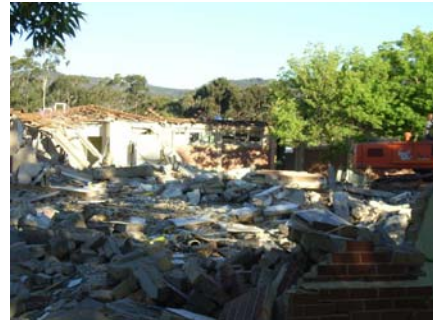
Demolition in progress at Magill.
