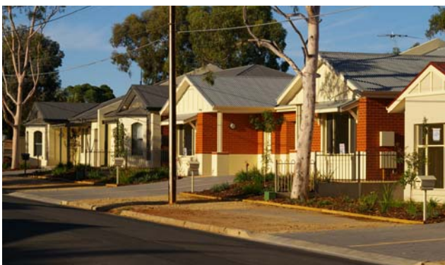
Units on Bricknell Street, Magill
